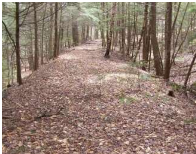
The raised railbed was laid on top of fill. It was not cut out of the hillside.
