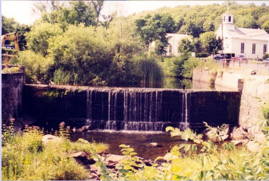
**Ballou Dam (1927)** Originally built in the 1800s for mill power, the 60-foot long, 14-foot high dam was reconstructed in 1927 after the dam was washed away during the flood. When it was rebuilt it provided water power to a basket factory located on Maple Street until the mid-1960's.
